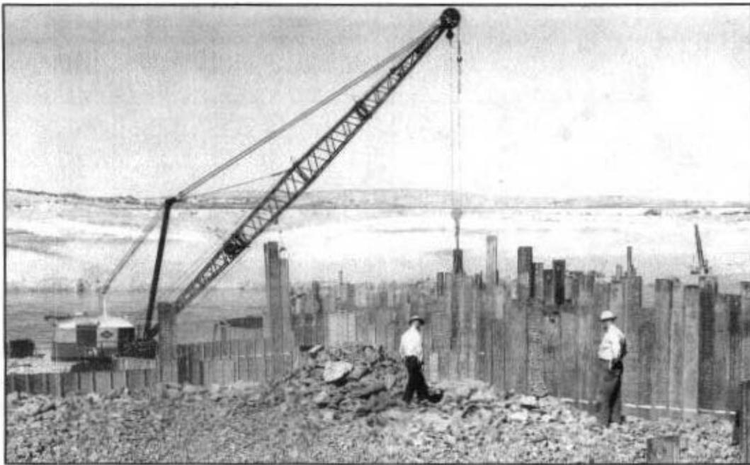
*Placing stone topping in the cofferdam cells, September 1956.*
